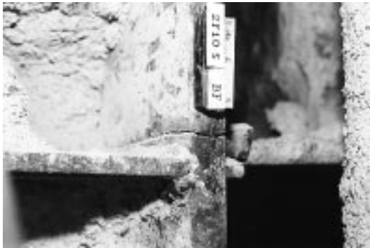
a. Fractures through Column Flange
