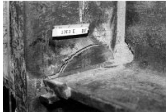
b. Column Flange "Divot" Fracture
