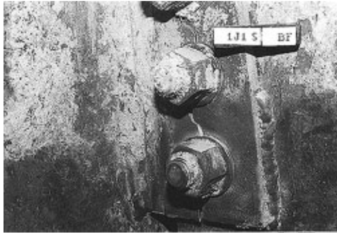
Figure 1-4 - Vertical Fracture through Beam Shear Plate Connection
