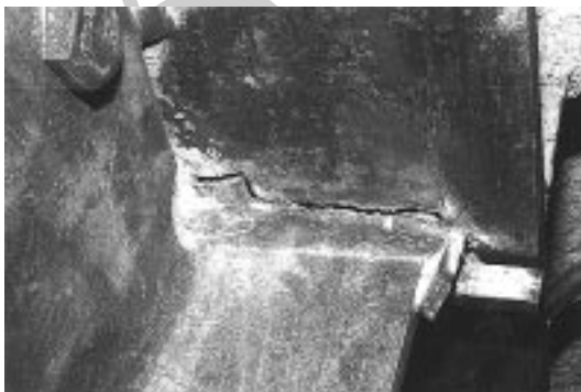
a. Fracture at Fused Zone
