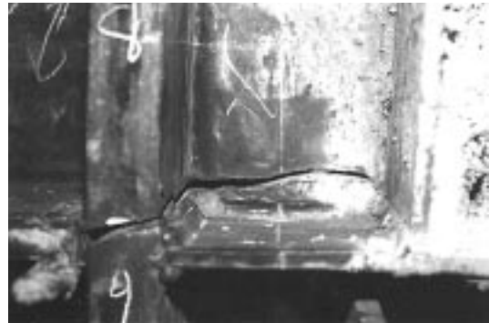
b. Fracture Progresses into Column Web
