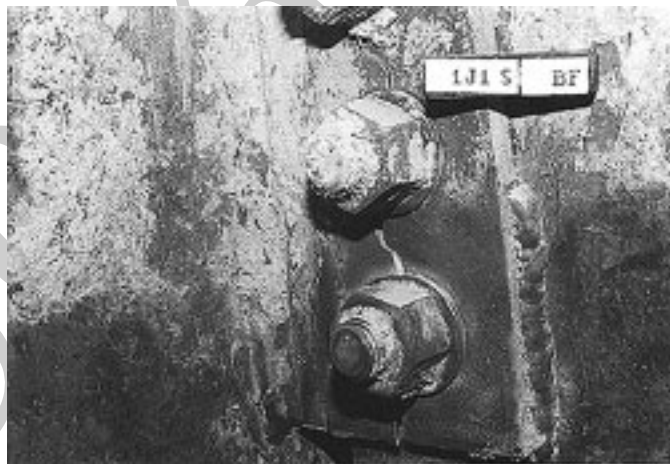
Figure 1-4 - Vertical Fracture through Beam Shear Plate Connection
