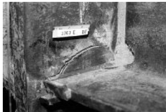
b. Column Flange “Divot” Fracture
