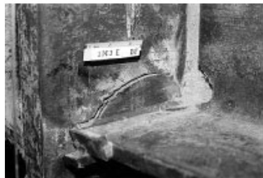
b. Column Flange "Divot" Fracture
