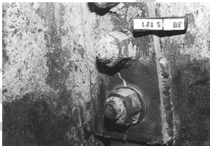
Figure 1-4 - Vertical Fracture through Beam Shear Plate Connection
